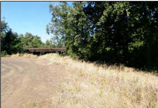
Looking north at Comanche Creek. Feature NJ 01b alongside vegetation break.
