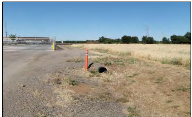
NJ 01a looking west where drainage enters culvert under the access road.
